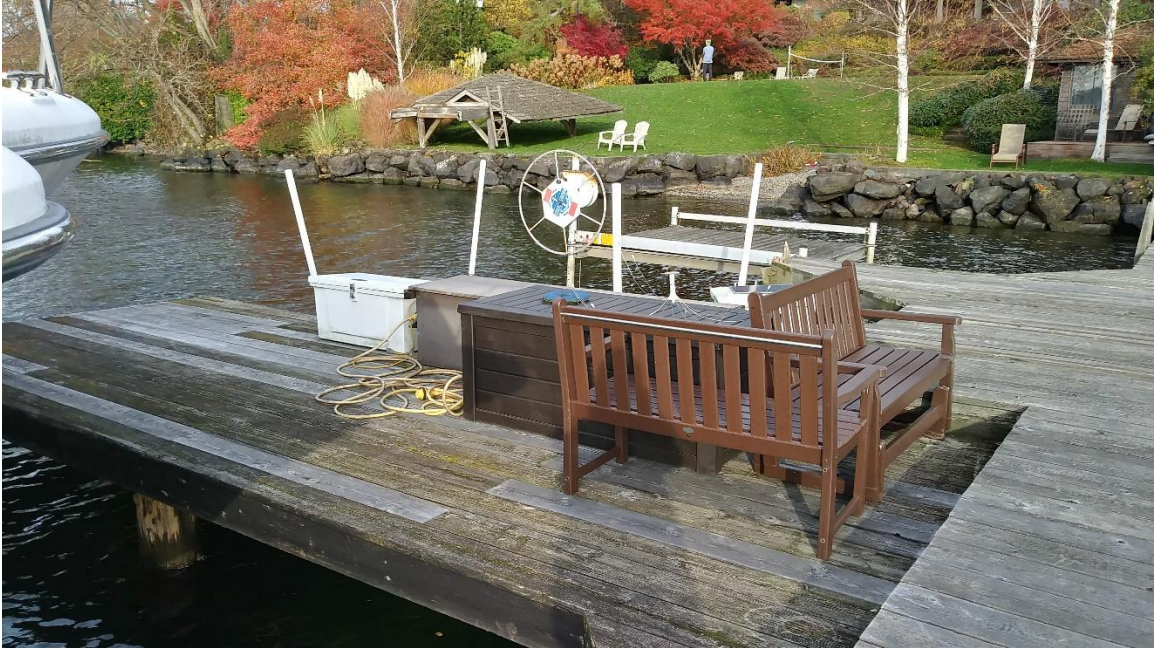
Photo 1. View of pier from southwest corner looking northwest.
